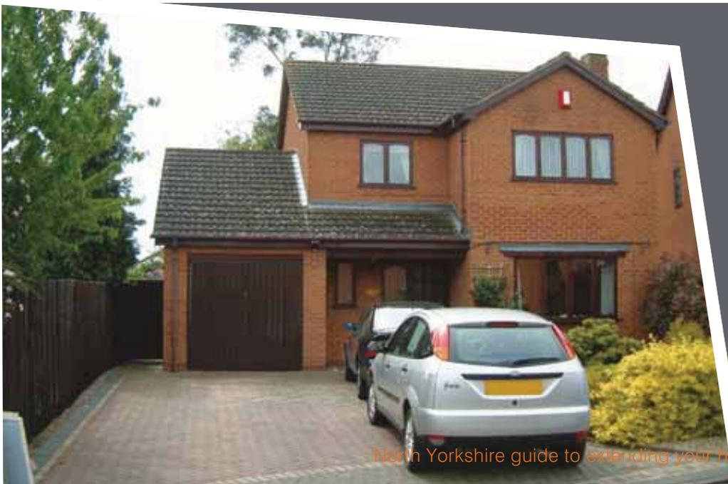
felt under them. The tiles are supported by the rafters via a series of timber battens. To provide adequate weather resistance the tiles overlap each other and they must have an adequate pitch. For extensions it is common to use tiles or slates that match the main house although this is not always possible if the extension roof has a very low pitch. Our Building Control Surveyors will be happy to assist you with any enquiries that you have about roof finishes.
